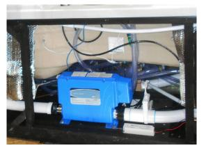
After the spa has been placed on an approved surface and has been correctly wired by a licensed electrician, inspect all plumbing connections in the equipment area of your spa. Ensure that these connections are secure and that they did not loosen during shipment.
