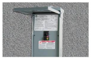
When the spa is filled to the correct level, turn on the power at the GFCI breaker. (Ensure that the 120V spas are connected to the proper electrical outlet.)
